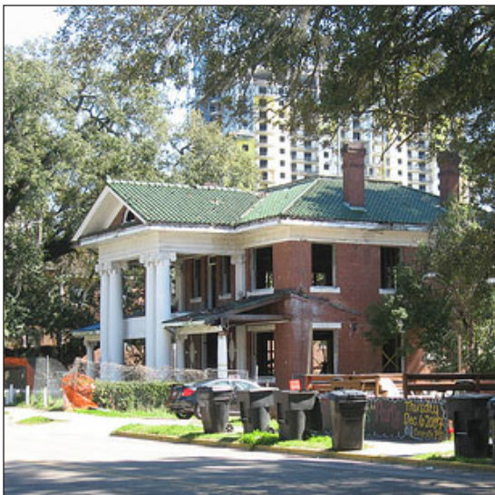
415 West College Avenue "Orion Parker House"
